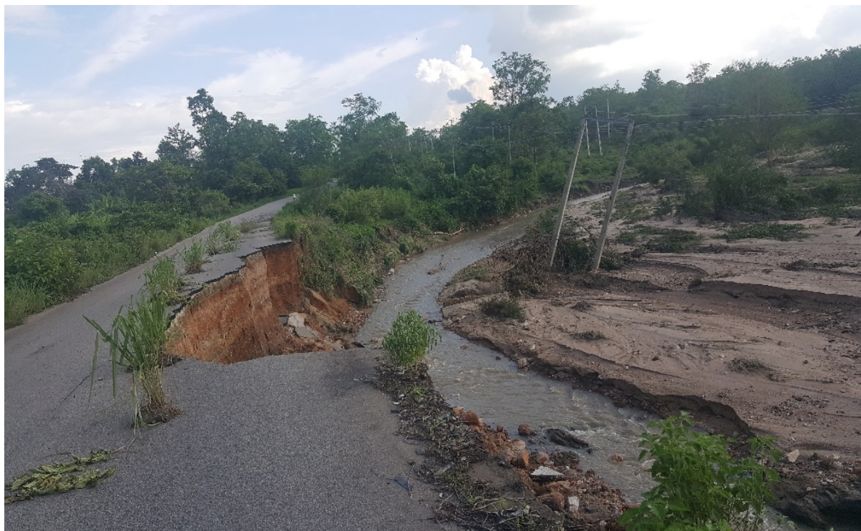
Plate 2: Road damaged by flood at Ajaokuta
